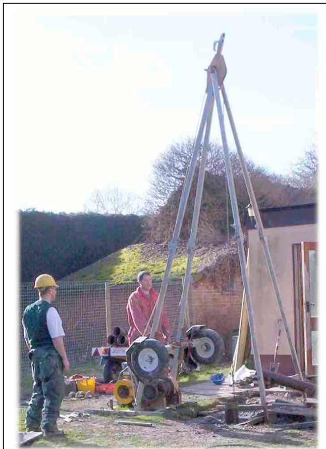
The Forager-55 cable percussion (Shell & Auger) rig shown here drilling in UK was powered by a 7½ hp diesel engine and operated by two men.
